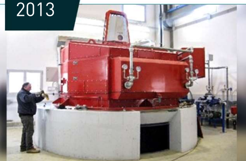
HPP CREMA 1200 kVA, 40P, 150 rpm, V1 - Onv 2660x275/40 Kaplan
