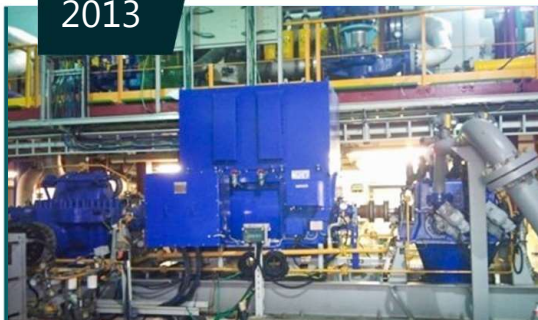
Via Maris Desalination Plant FTA Type MV Motors (9x 315 kW-5000 kW)
