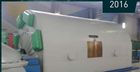
JAVNO PODJETJE ENERGETICA LJUBLJANA D.O.O., Slovenia NEW stator together with rotor refurbishment KONCAR make, Type: S-1925-2, 49.5 MVA, 10500 V, 50 Hz, 2 poles
