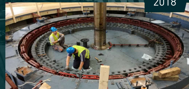
Granfors Hydro Power Plant, Sweden Stator manufacturing & rotor refurbishment of ASEA GS 2910 type 25 MW, 150 rpm generator.
