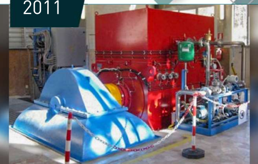
HPP COGNO, Italy 3x 2400 kVA, 6P - SRGb 636Ks6 Pelton
