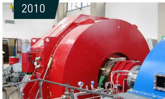
HPP Albano, Italy FVM 909E14 (1200 kW, 11000 V, 424 rpm)
