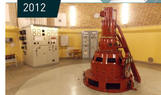
HPP Gavünda, FORTUM Sweden 9000 kVA 250 rpm Kaplan Vertical
