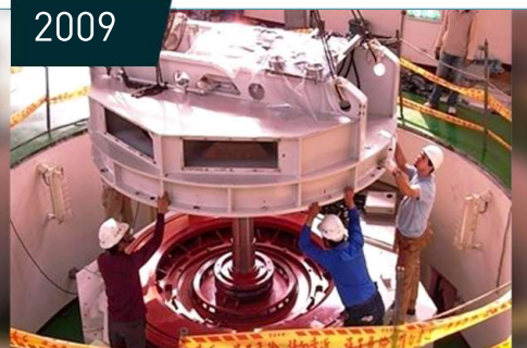
HPP Zho Tuwei, Taiwan 4000 kVA, 30 pole, V1 ONv2600L30 Kaplan
